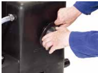
密封圈安装 Lip seal Installation
